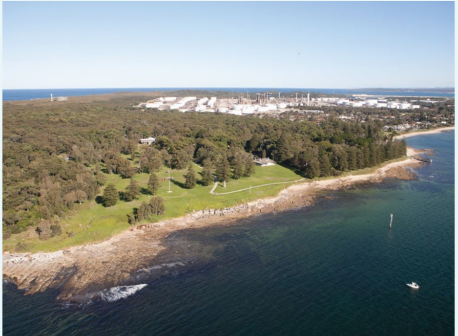
The Kurnell peninsula, Sydney, the site of Caltex's refinery for almost six decades, now features Australia's largest fuel import terminal.
