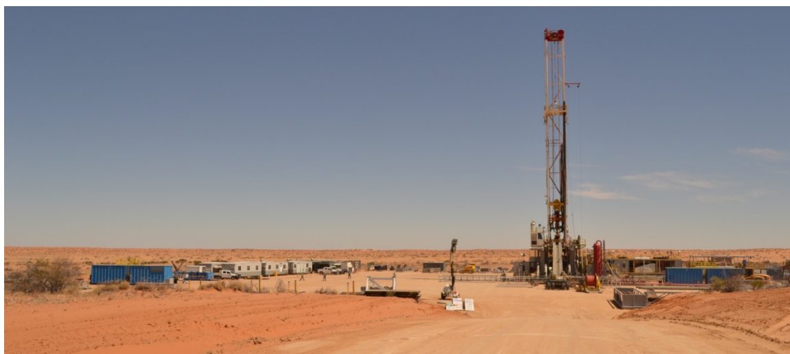
Drilling at Spinel-1 in PEL 513
