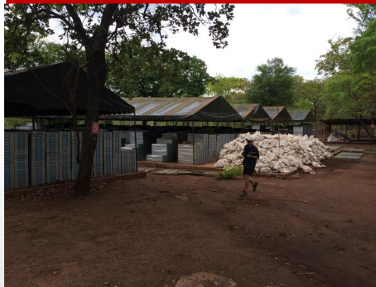
Core Storage Sheds
