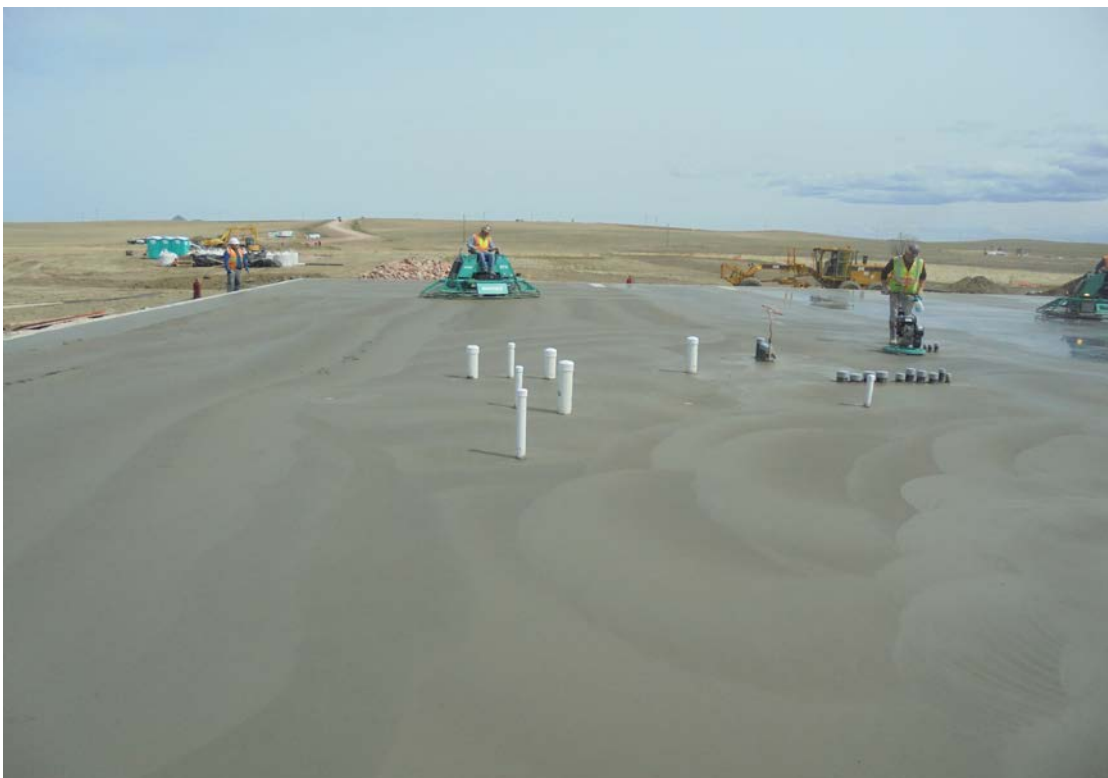
Figure 3: Administration Building concrete slab
