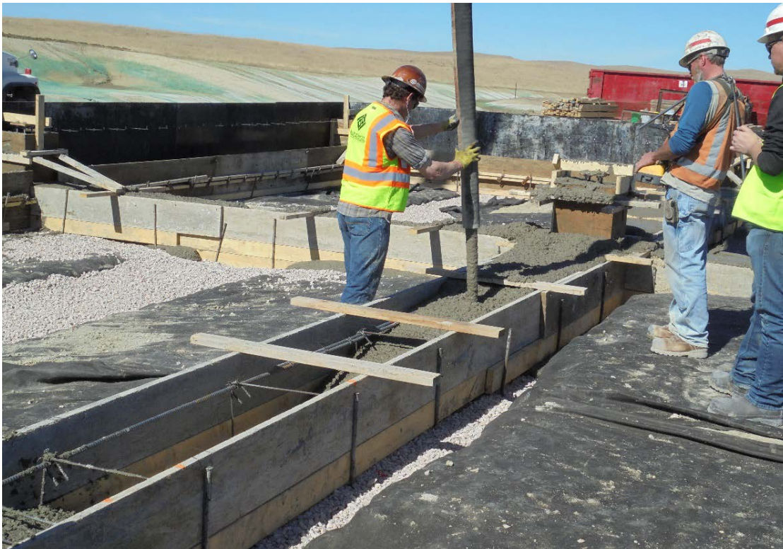
Figure 2: Pouring of foundations for CPP
