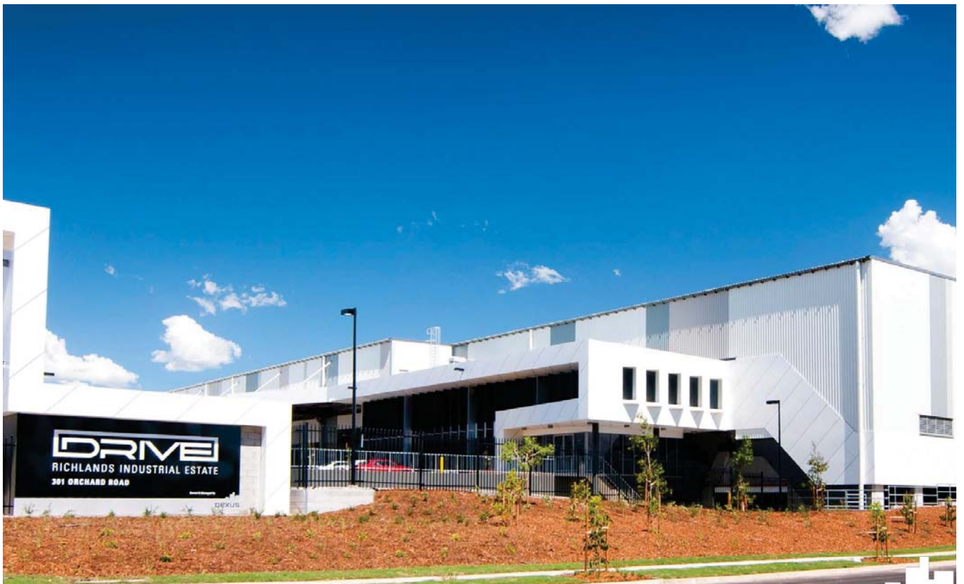
Drive Industrial Estate, Richlands in Brisbane, a DWPf development.
