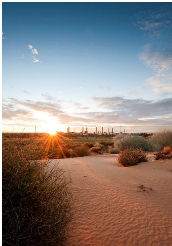
Moomba Plant, Cooper Basin
