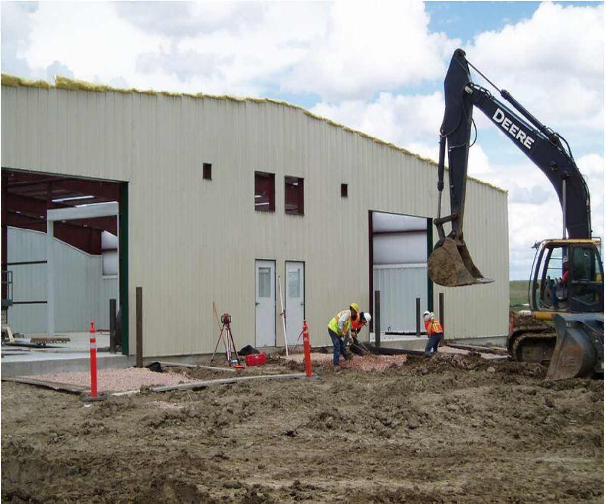
Figure 4: External finishing activities in progress at site workshop and administration building
