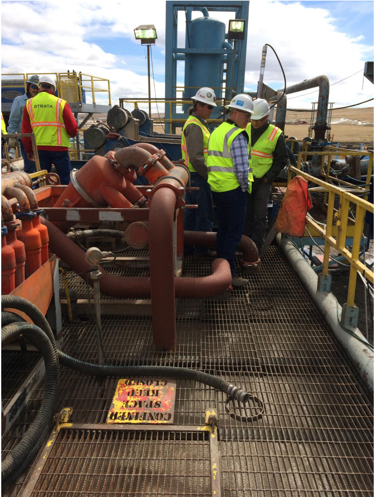
Figure 2: DDW drilling rig operational observation platform
