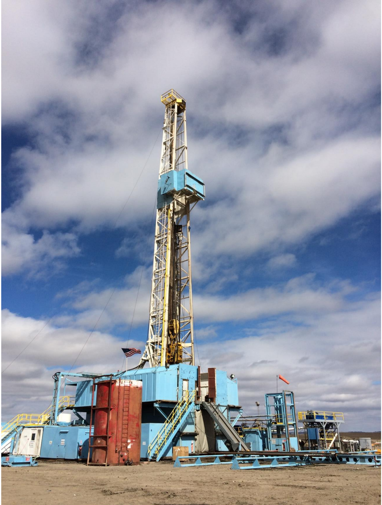
Figure 1: Deep Disposal Well drilling rig
