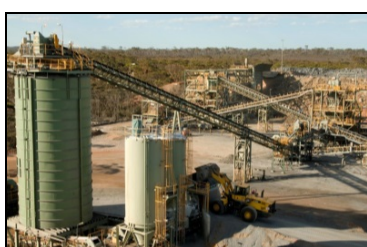
Lake Johnston Processing Plant
