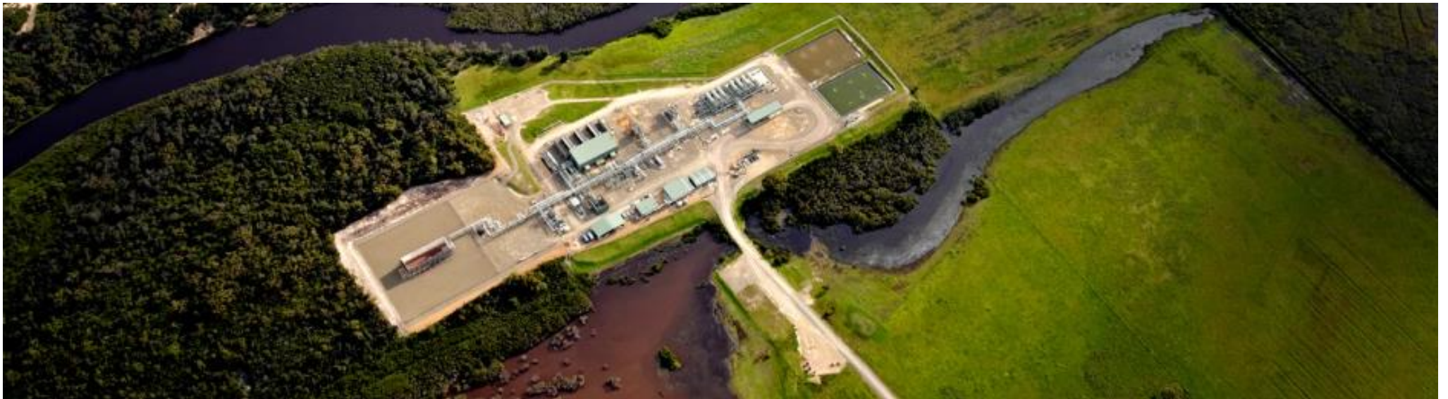
Orbost Gas Plant, Cooper Energy interest 50%
