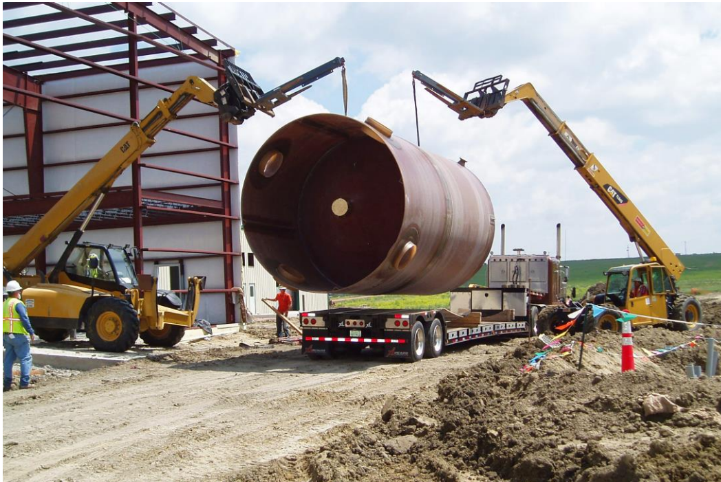
Figure 1: Unloading of tanks at the CPP
