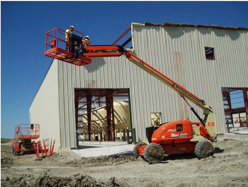
Figure 3: External cladding being fitted to CPP Building
