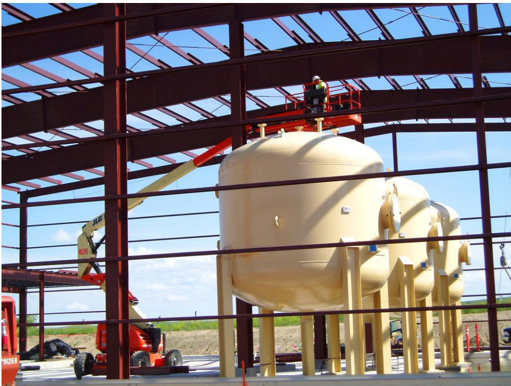
Figure 2: Ion Exchange Columns within the CPP
