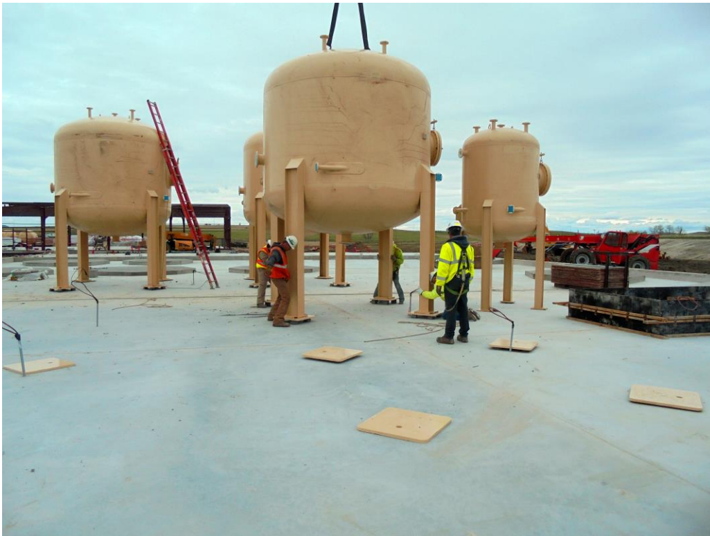
Figure 1: Ion Exchange Columns being installed on site
