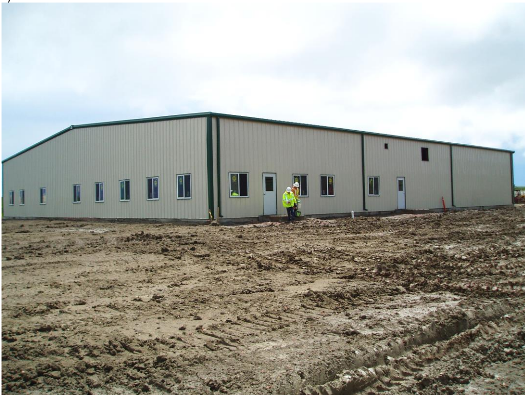
Figure 4: Administration and Workshop Building
