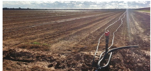
Installation of drip tube irrigation prior to planting
