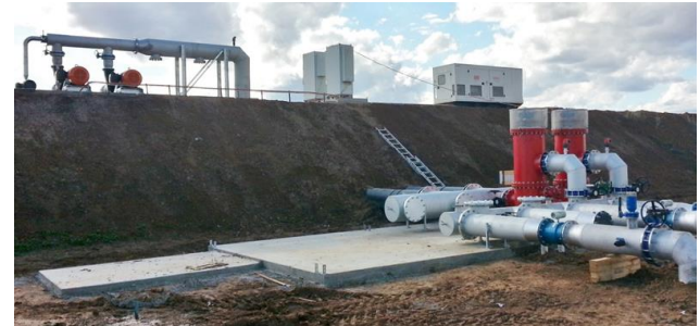
Pump station under construction
