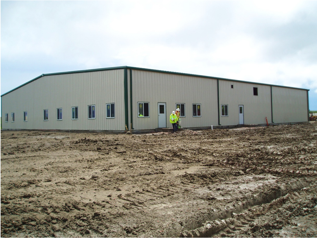
Figure 2: Administration and Workshop Building, Wyoming, USA
