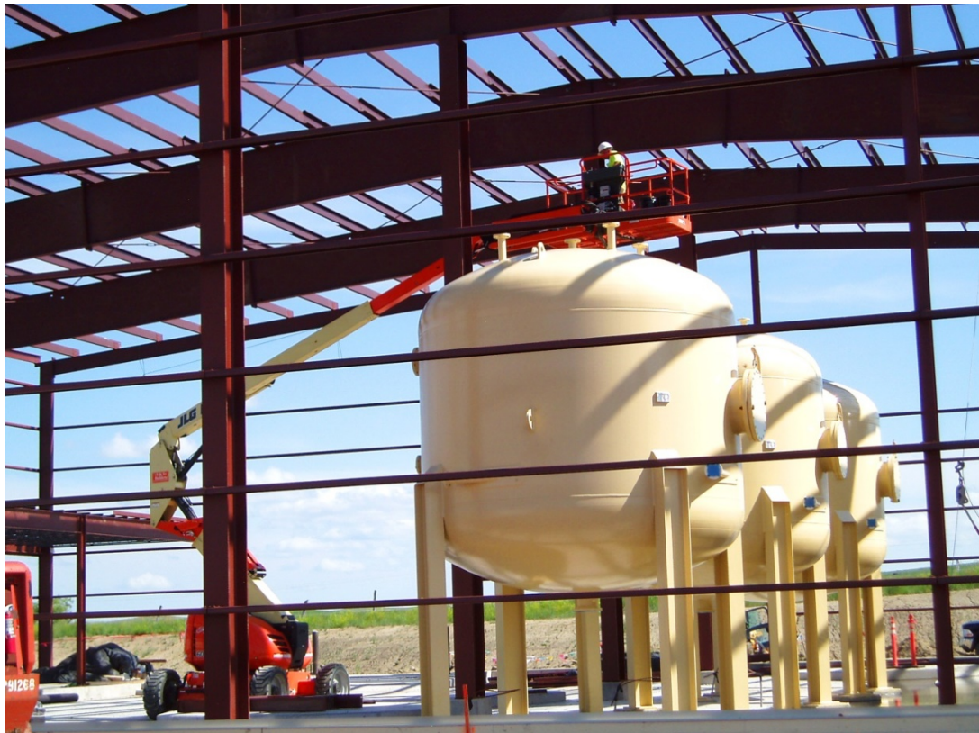
Figure 3: Ion Exchange Columns being installed within the CPP, Wyoming USA
