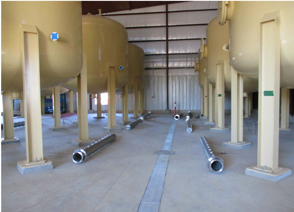
Figure 4: Completed Ion Exchange Columns within the CPP, Wyoming USA
