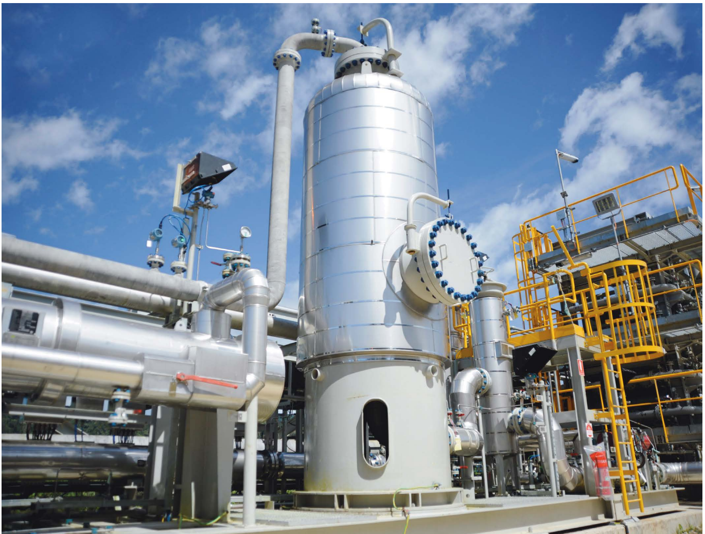
Top Resource Estimator Aaron Brown working at the Dehydration Bed at Karratha Gas Plant, Karratha, Western Australia
