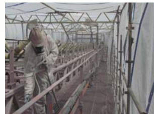
Protective Coatings (Blast & Paint)
