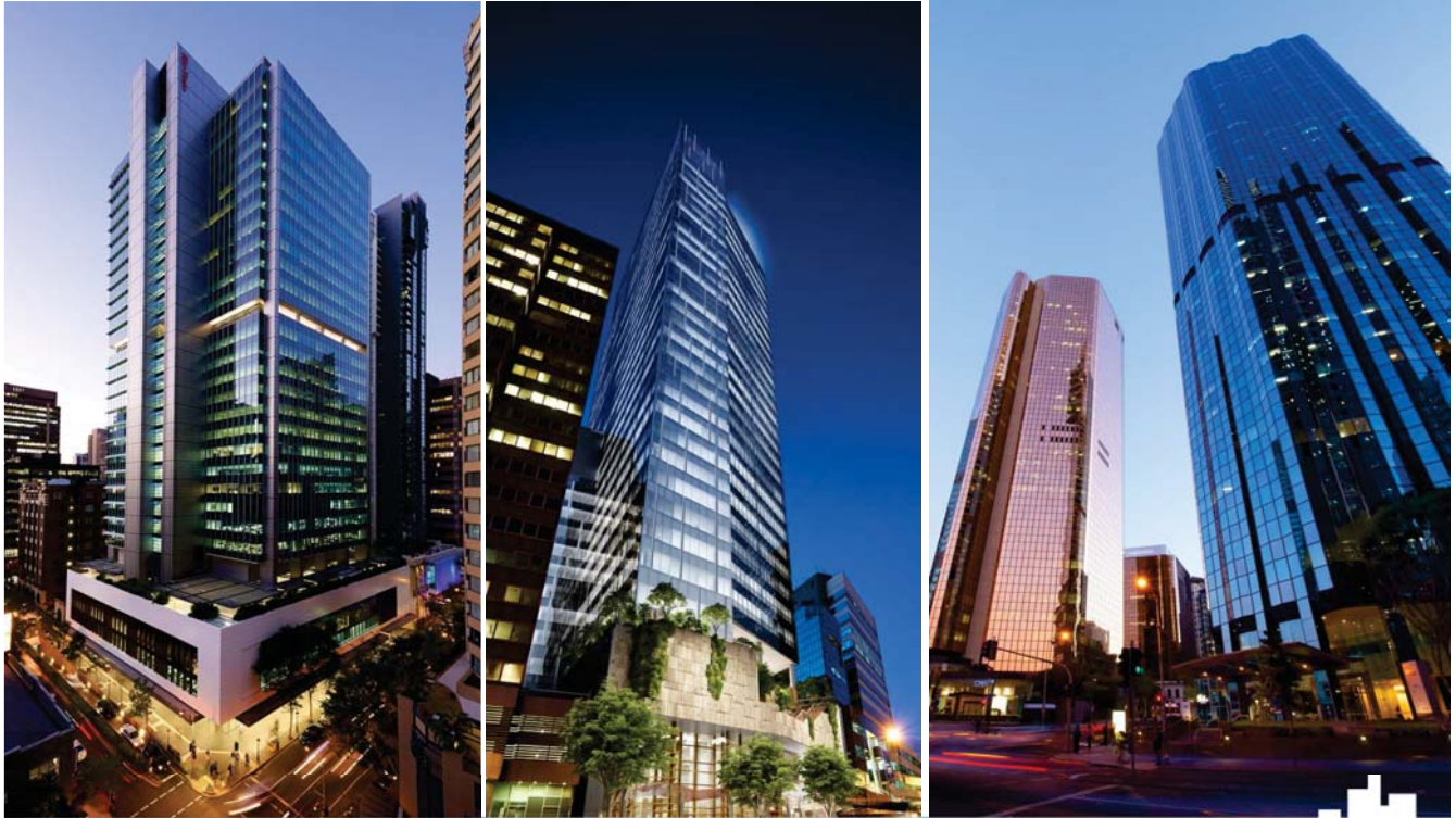
L-R: 123 Albert Street, 480 Queen Street development, 10 Eagle Street and 12 Creek Street, Brisbane, QLD.
