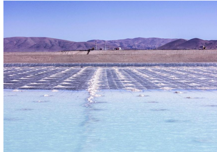
Empty Evaporation Pond
