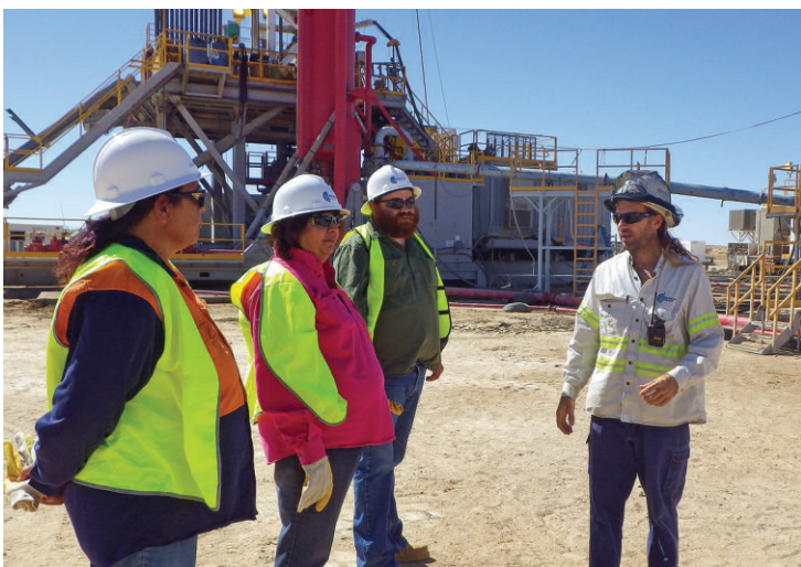
Beach Drilling Supervisor Michael Thompson (Far right), providing a tour of Rig 965 to the Dieri survey team (L-R) Mandy Tuipuloto, Leanne Warren and David Strangways.
