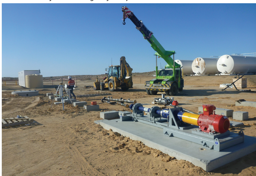
Construction of the Pennington facility
