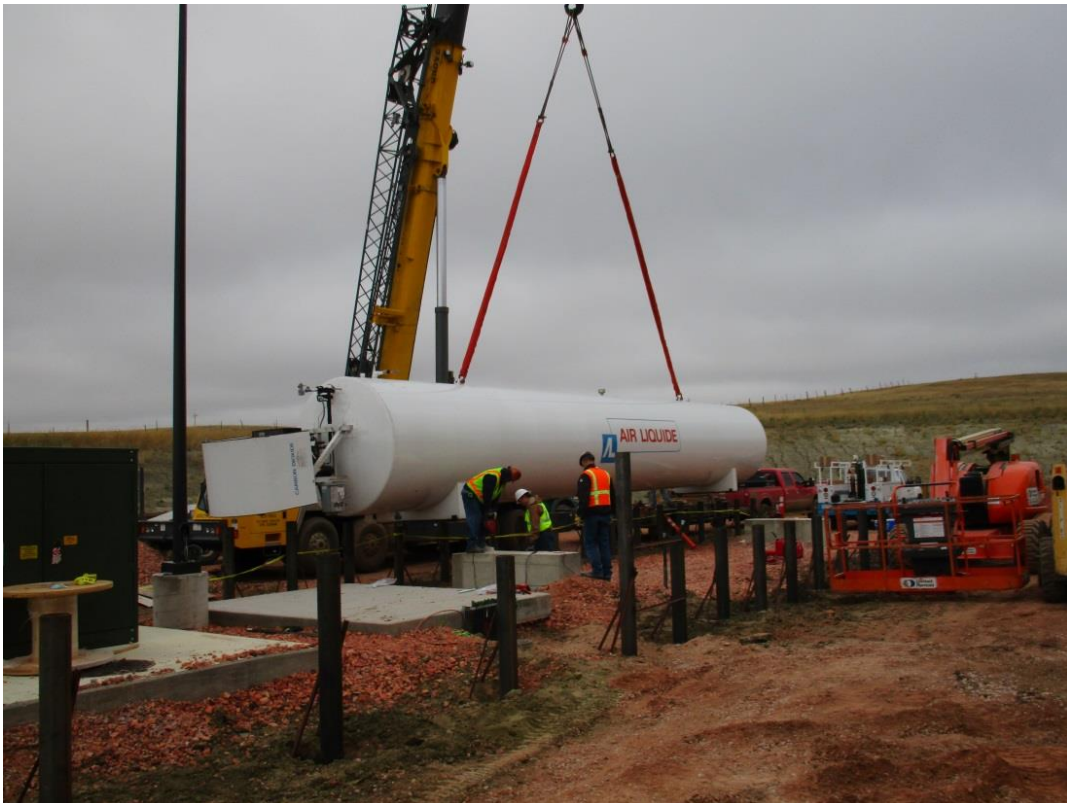
Figure 6: Installation of Carbon Dioxide tank at the CPP Lance Projects – 29 September 2015
