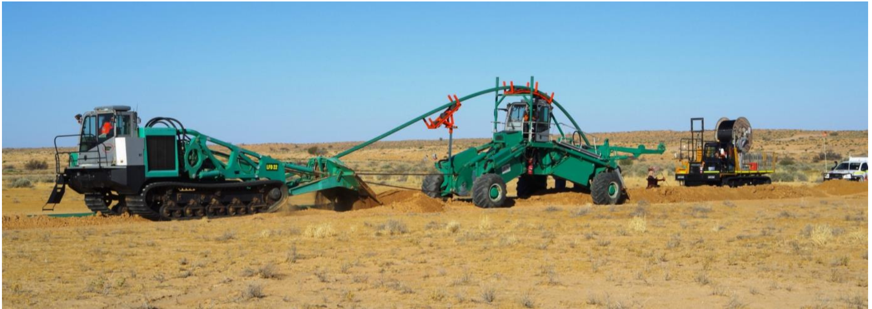
Installation of Stunsail to Bauer oil pipeline with direct plough technique
