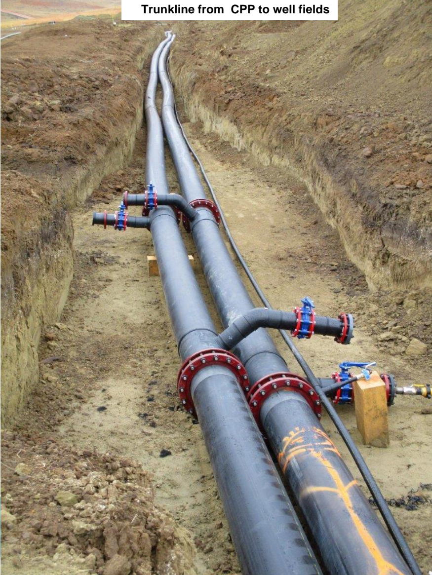
Trunkline from CPP to well fields
