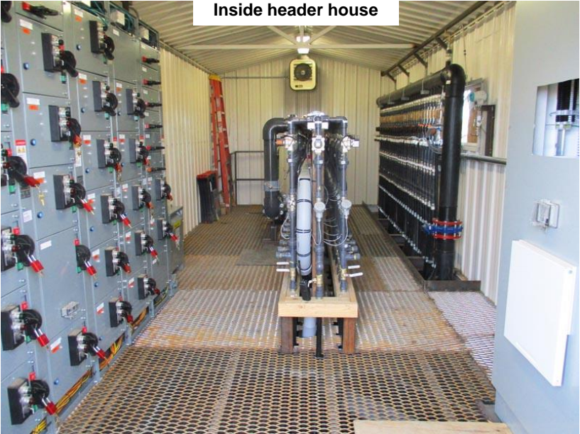
Oxygen Injection System
