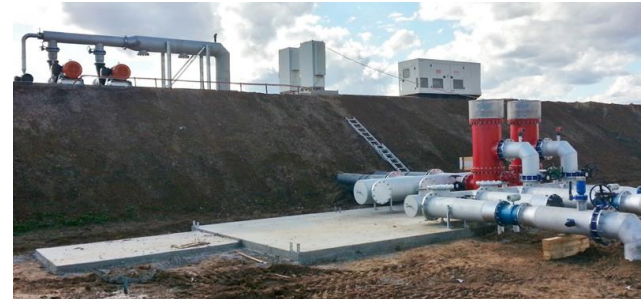
Pump station under construction
