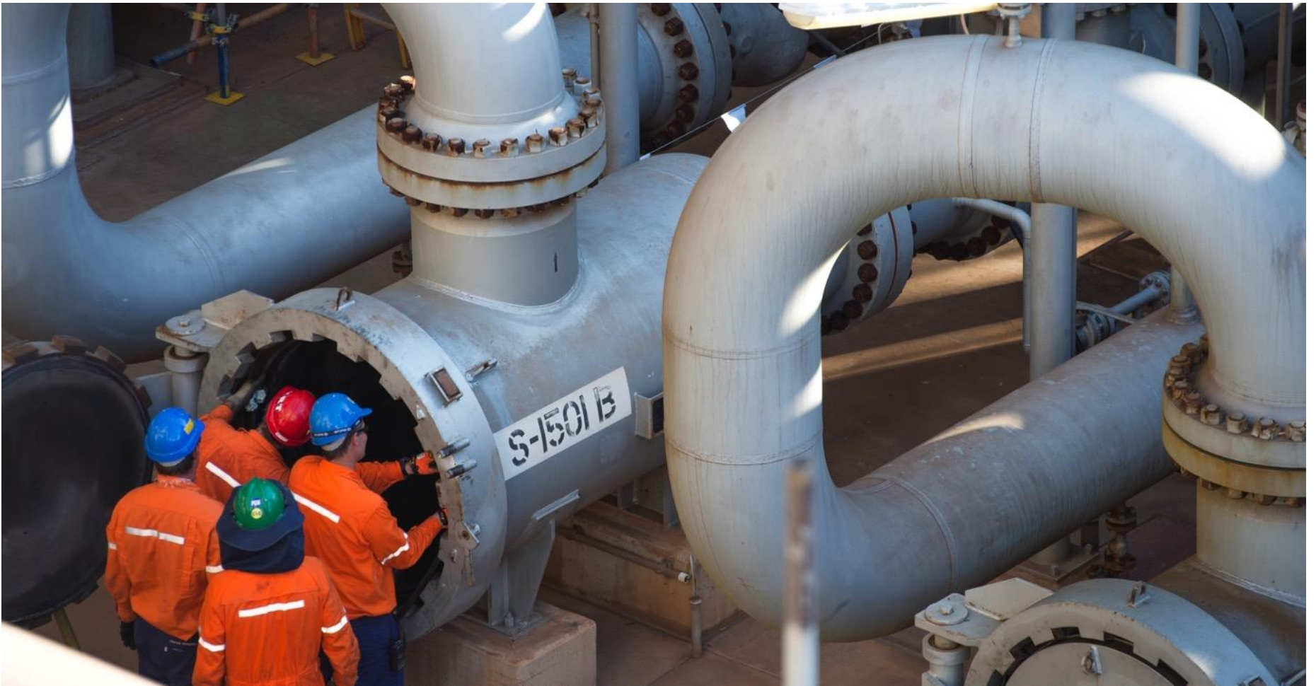
Woodside, Karratha Gas Plant, Karratha, Western Australia
