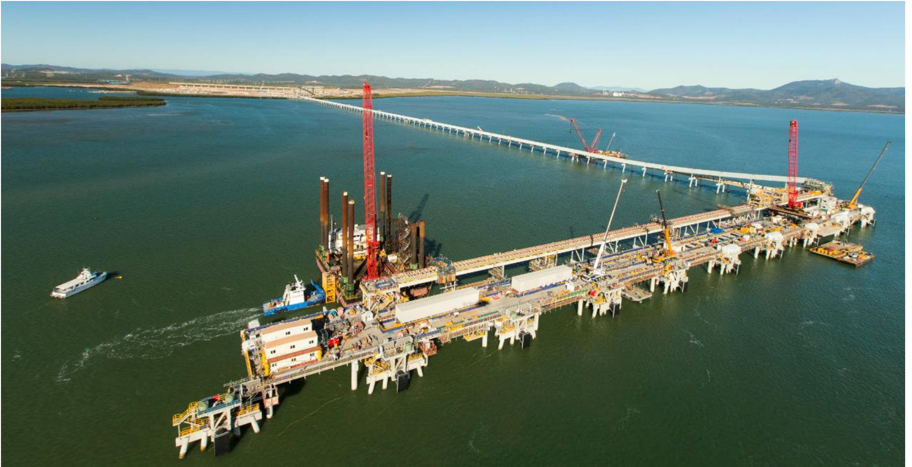
Wiggins Island Coal Export Terminal, Gladstone, Queensland
