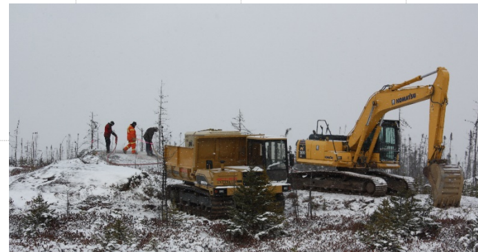
James Bay earth-moving equipment
