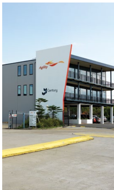
2-4 Military Road, Matraville NSW
