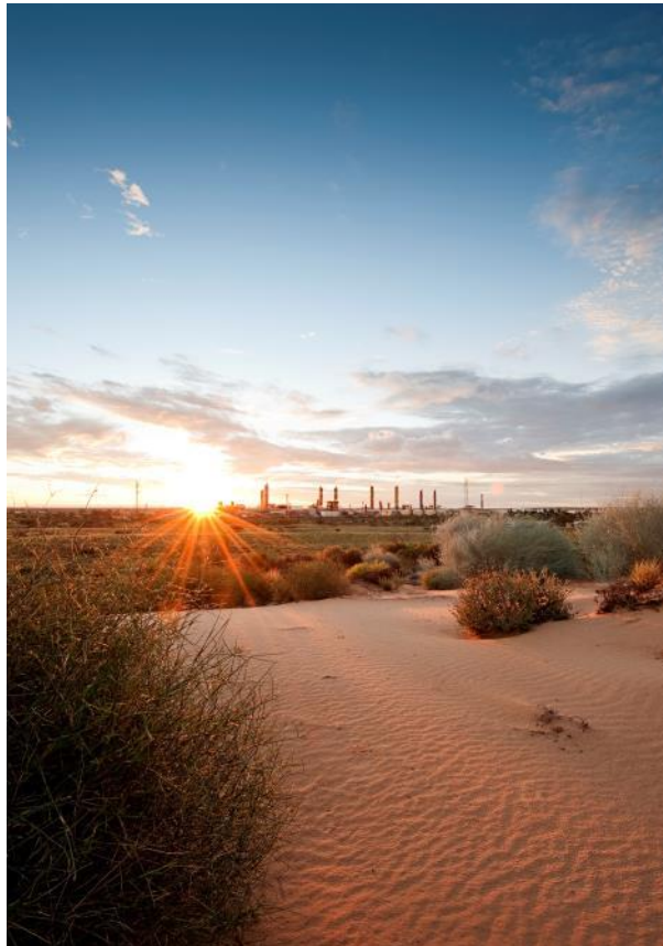
Moomba Plant, Cooper Basin
