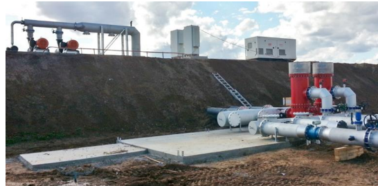
Pump station under construction
