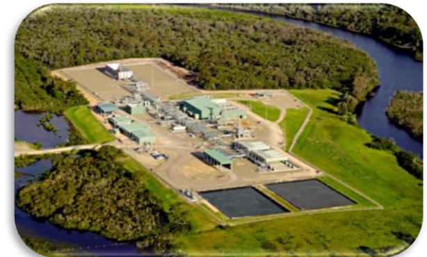
Orbest Gas Plant
