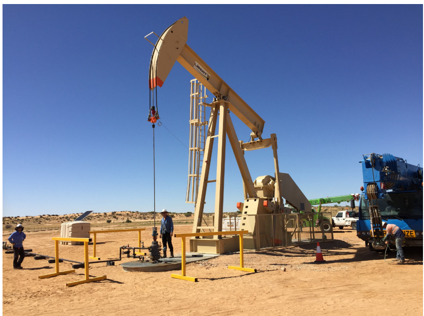
Construction of the Kalladeina-2 beam pump
