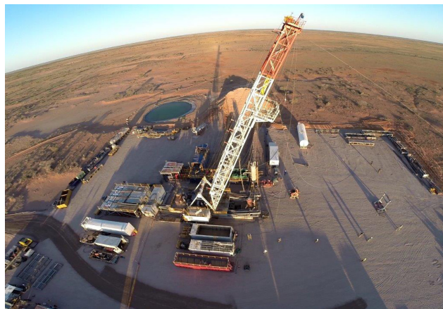
Raising the drill mast at Maroochydore-1
