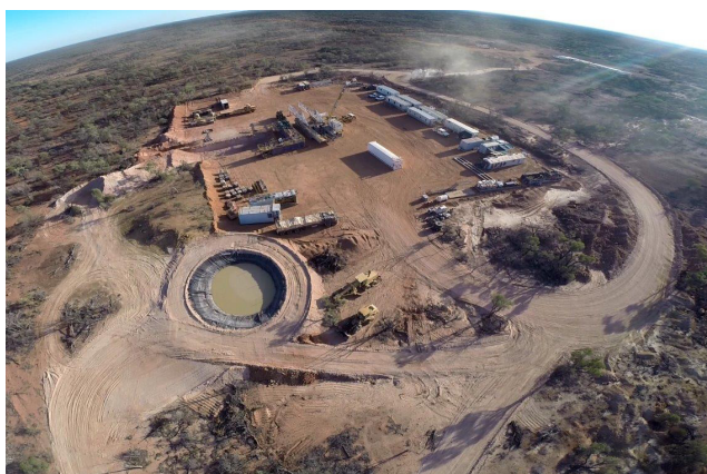
Setting up for drilling at Thylungra-2
