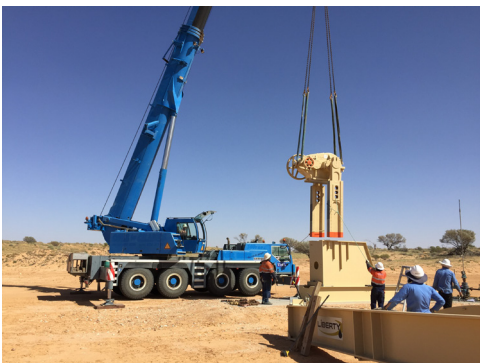
Construction of the Kalladeina-2 beam pump
