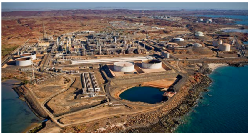
Woodside-operated Karratha Gas Plant, North West Shelf Project.
