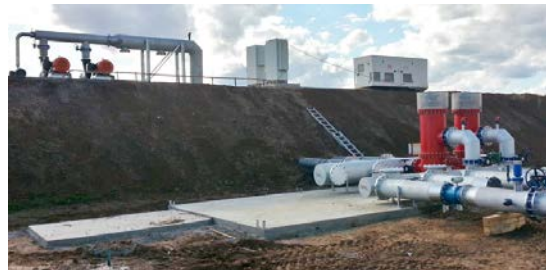
Pump station under construction
