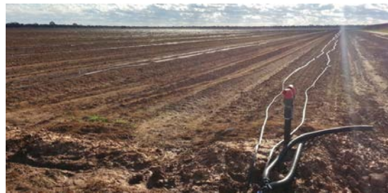
Installation of drip tube irrigation prior to planting
