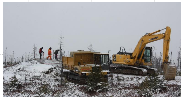
James Bay earth-moving equipment
