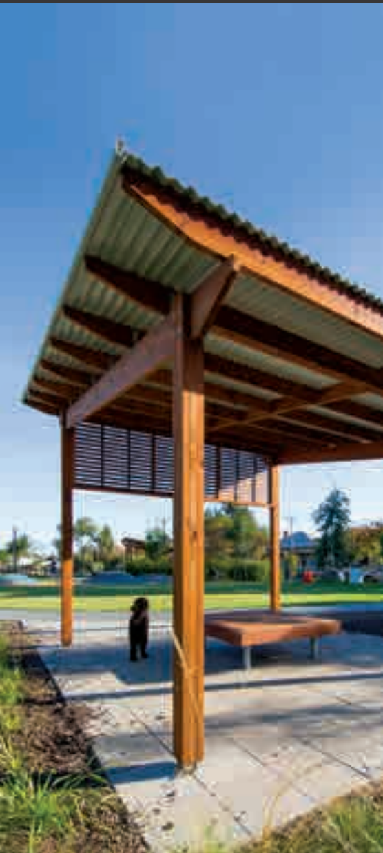
Public multi-purpose community park adjacent to the Birkenhead plant constructed by Adelaide Brighton Cement
