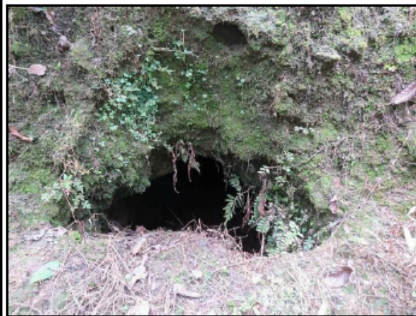
Adit filled with debris – Location No.5
