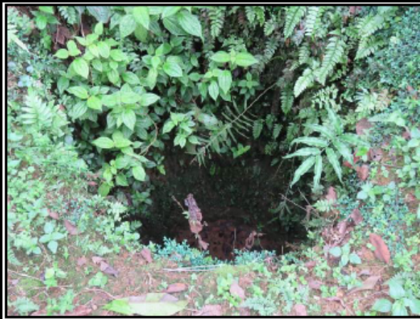
Ventilation Shaft - Location No 1
