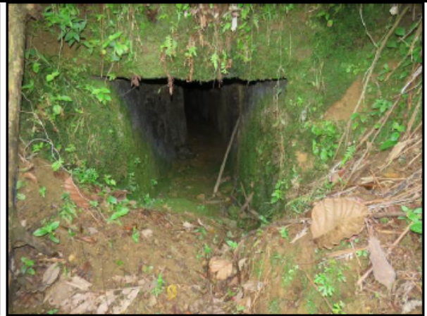
Adit - Location No.4
