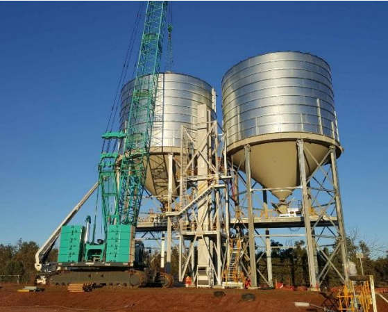
New over-rail bins and siding Calleen, SNSW
