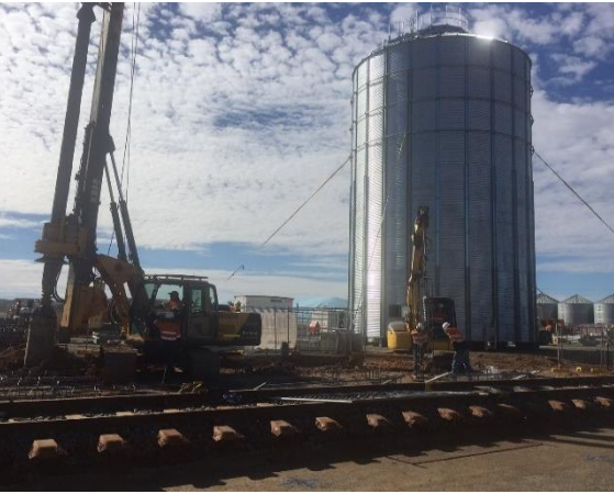
New over-rail bins and siding Ardlethan, SNSW
