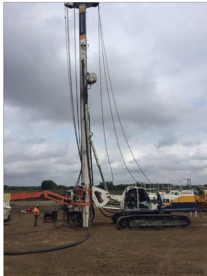
INITIAL DRILLING FOR GRAIN ELEVATOR CONSTRUCTION AT MAYMONT, SASKATCHEWAN
