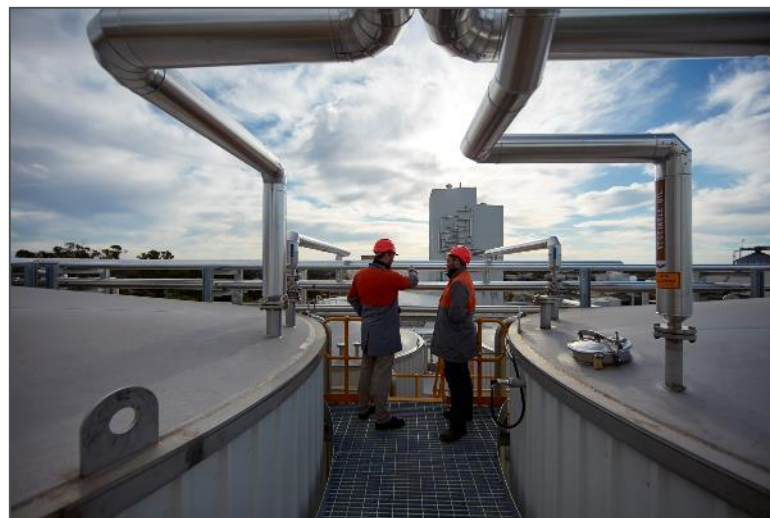
NUMURKAH SITE UNDER CONSTRUCTION FOR OPTIMISATION PROJECT
