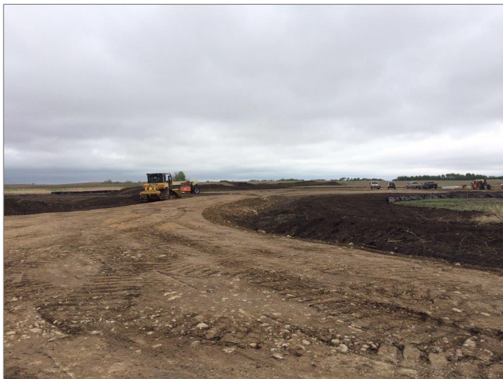
SITE PREPARATION AT MAYMONT, SASKATCHEWAN
