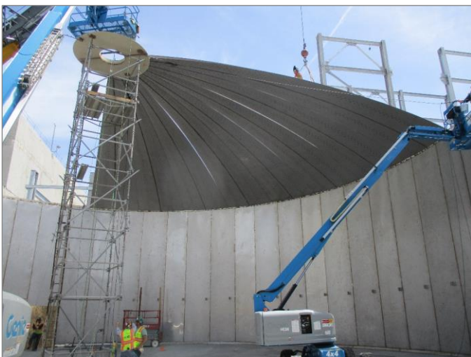
GERMINATION BED ROOF BEING ASSEMBLED
