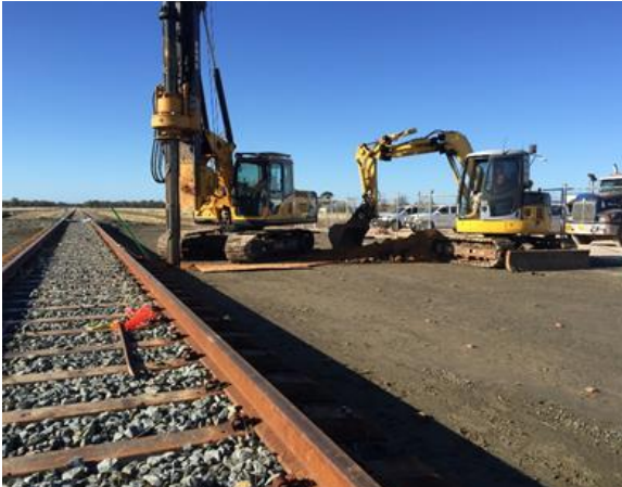
New over-rail bins and siding Nevertire, NNSW
