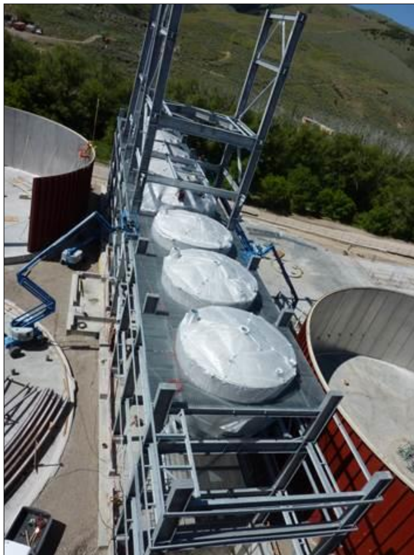
STEEP TANKS IN PLACE
