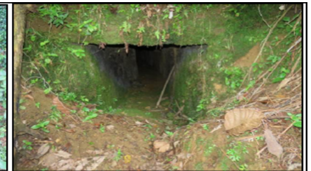
Adit - Location No.4
