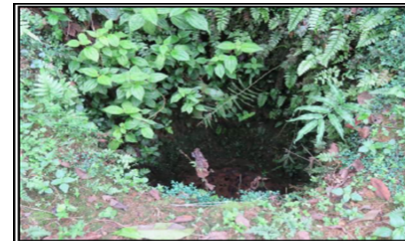
Ventilation Shaft - Location No 1
