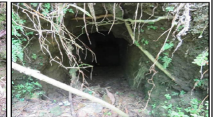
Adit – Location No. 6
