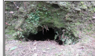
Adit filled with debris – Location No.5
