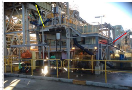
Fig. 3: Stockpiling of feed for DMS circuit after tantalum removal
