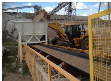
Fig. 1: Front end loader tipping on to Feeder 07, bypassing the crushing circuit
