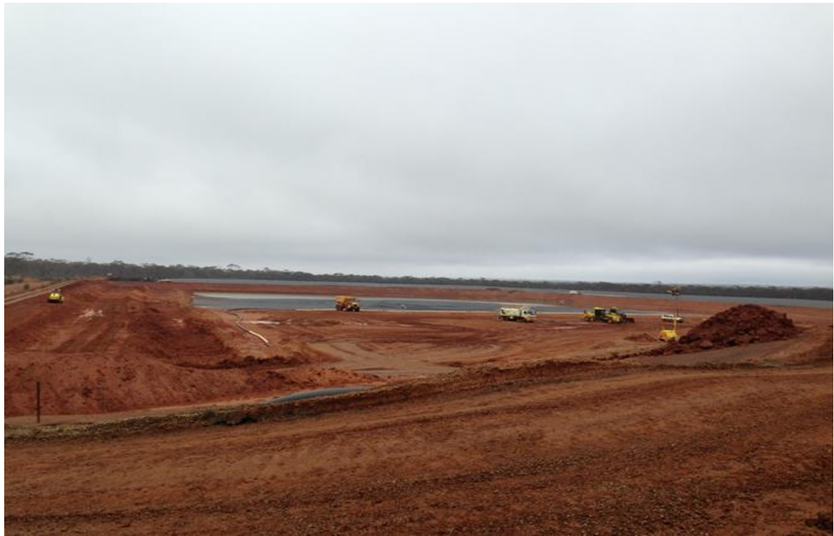
Figure 4: Tailings Disposal Cells at Lake Johnston
