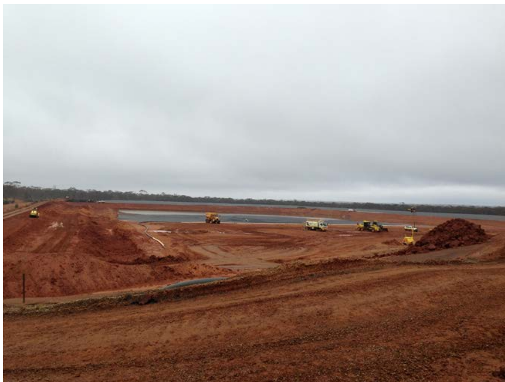
Figure 5: Tailings Disposal Cells at Lake Johnston
