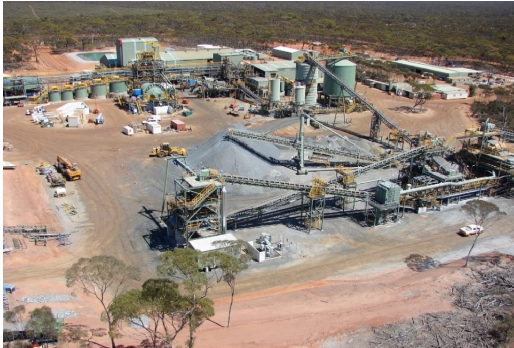
Figure 4: Lake Johnston 1.5MTPA Process Plant
