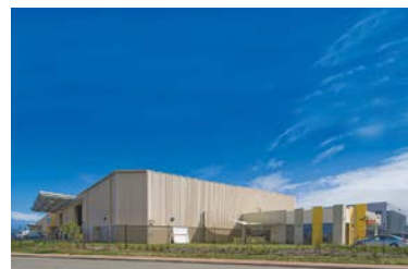
5 Butler Boulevard, Adelaide Airport
