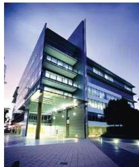
Building C, 1 Homebush Bay Drive, Rhodes
