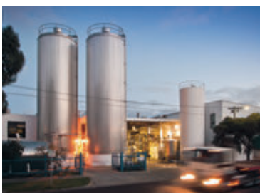
COBURG 10-16 Allenby Street Coburg VIC 3058 Australia
