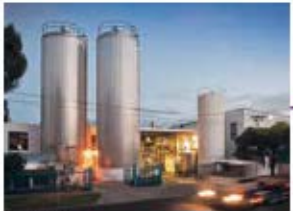
COBURG 10-16 Allenby Street Coburg VIC 3058 Australia
