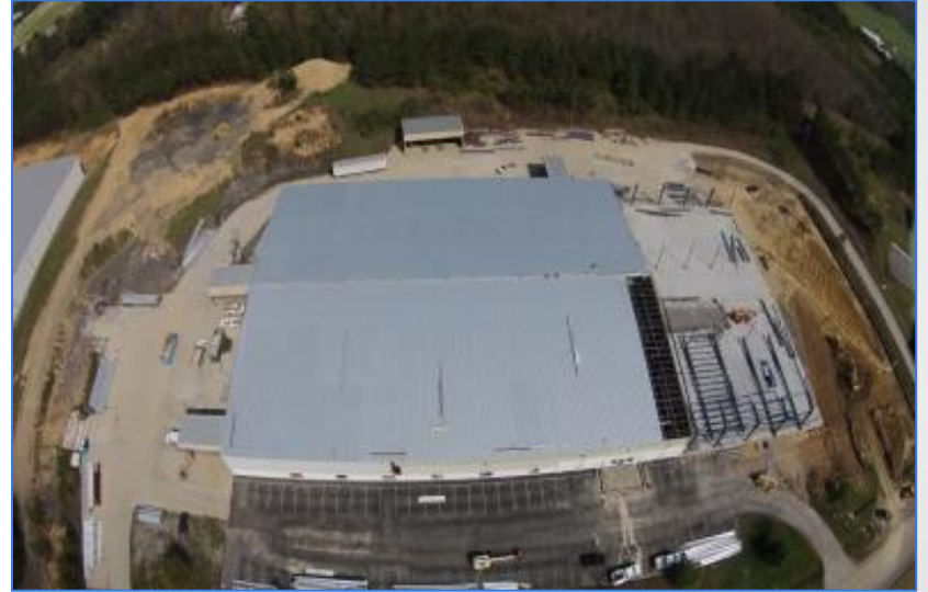
Additional Expansion on the South of the Building
