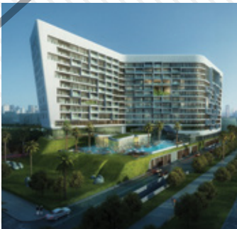
RAPID P1 CAMP by EPCC Contractor CCSM, Synerlitz (Malaysia) Sdn Bhd
