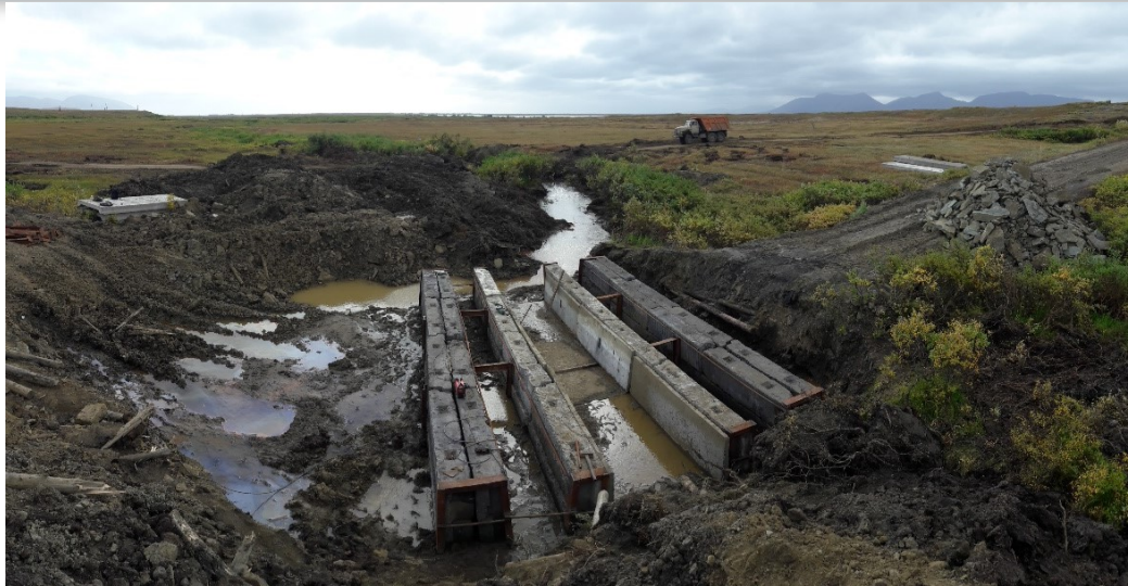
Construction of culverts and stream crossings
