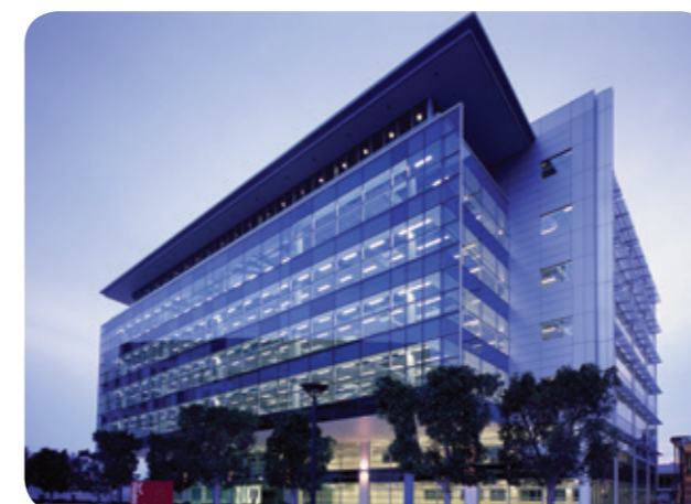
Building A, 1 Homebush Bay Drive, Rhodes
