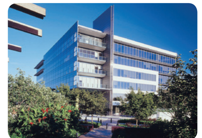
Building C, 1 Homebush Bay Drive, Rhodes
