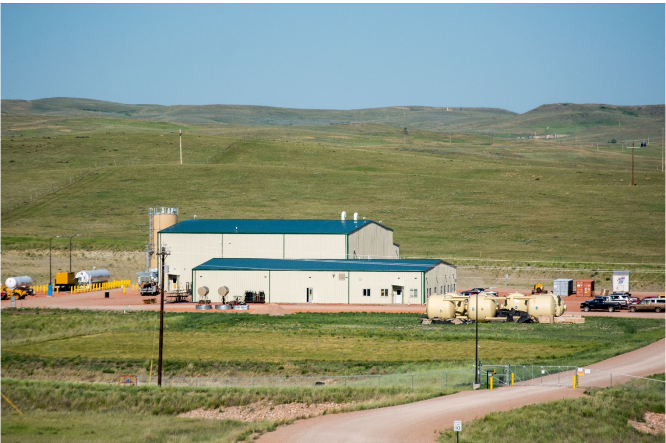
Figure 2: CPP and Admin Building, Lance Projects, Wyoming USA – June 2016
