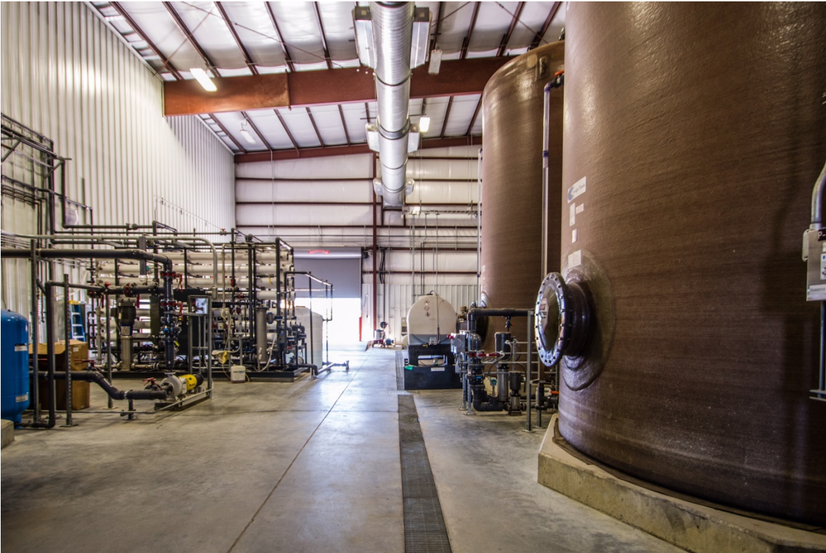
Figure 5: Inside CPP, Lance Projects – June 2016
