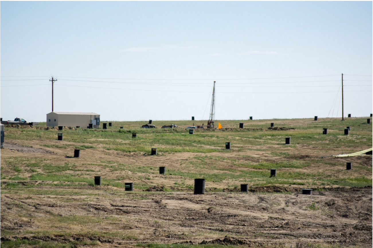
Figure 3: Well fields (and header house), Lance Projects – June 2016
