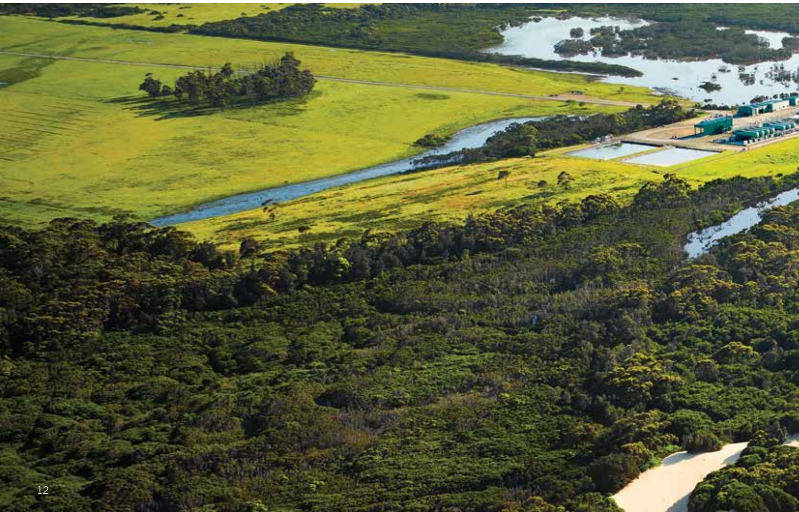
Orbost Gas Plant
