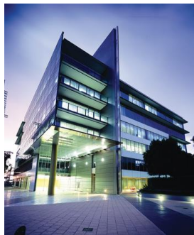
Building C, 1 Homebush Bay Drive, Rhodes
