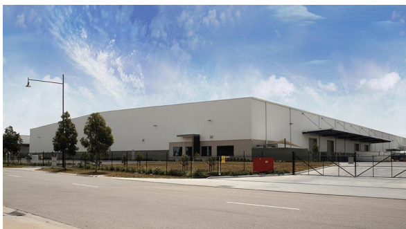
80-96 South Park Drive, Dandenong South
